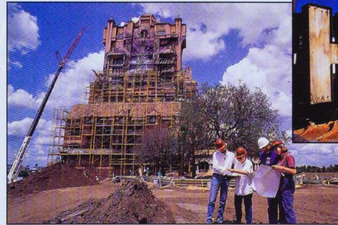
Show Producer Laine Akiyama (second from left) reviews plans with other Imagineers while the still-scaffolded Hollywood Tower Hotel looms in the background.
